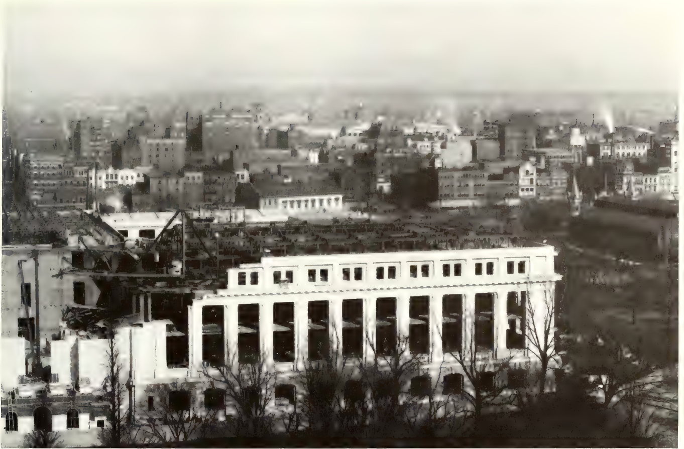
Construction of the east wing to the third-floor level and the rotunda to the fourth-floor (attic) level; probably taken in 1907 from the tower of the Castle. In the middle distance is the Old Patent Office building, the current site of the National Museum of American Art and the National Portrait Gallery.
